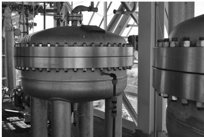
Figure 5. \text{CO}_2 absorbers.
