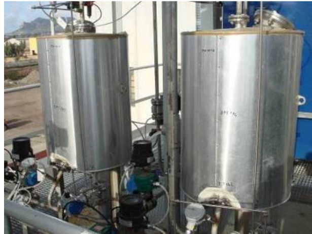
Figure 4. Hot gas desulphurization system.
