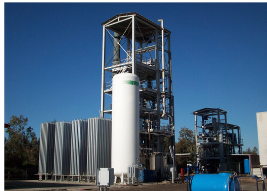
Figure 1. The Sotacarbo pilot platform.
